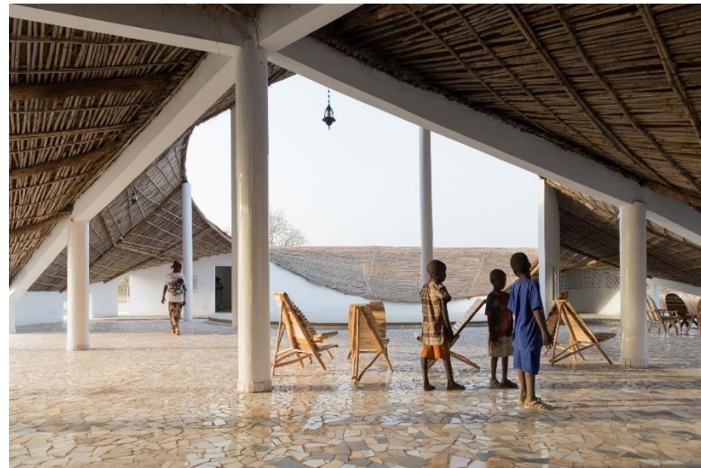
Figura 4.44: Pavimento in piastrelle rotte. Fass School and Teachers' Residence, Toshiko Mori, Fass, Senegal, 2019 (fonte: dezeen, https://www.dezeen.com/2017/01/25/toshiko-mori-compressed-earth-bamboo-thatch-cultural-centre-senegal-africa-architecture/ , ultima consultazione 18/08/2023)
