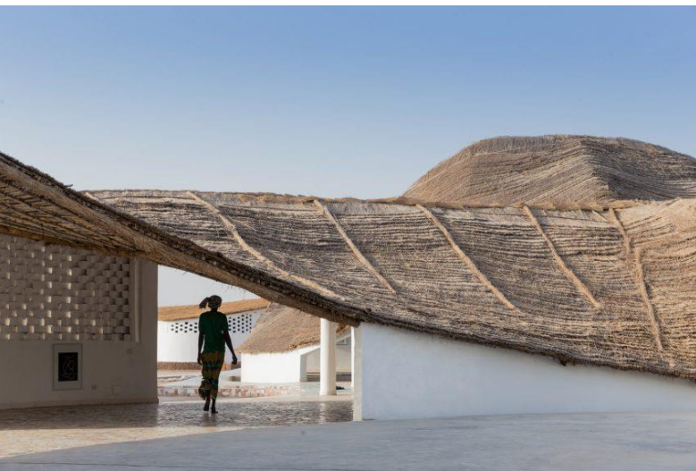
Figura 4.43: Copertura in fibre vegetali Fass School and Teachers' Residence, Toshiko Mori, Fass, Senegal, 2019 (fonte: dezeen, https://www.dezeen.com/2017/01/25/toshiko-mori-compressed-earth-bamboo-thatch-cultural-centre-senegal-africa-architecture/ , ultima consultazione 18/08/2023)
