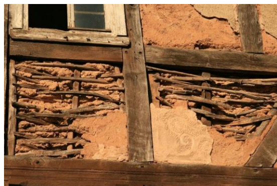
Figura 4.36 Tecnica del Wattle and daub. (fonte: GeeFix, https://www.geefix.com/wattle-and-daub/ , ultima consultazione 18/08/2023)
