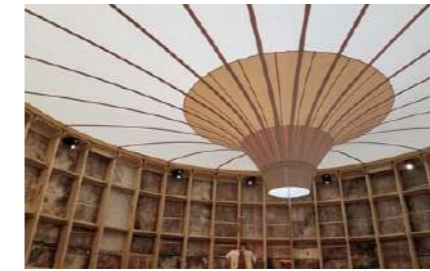
Figure 05.8.5: Growing pavilion - (NL) - EcoHemp roof Source: https://thegrowingpavilion.com
