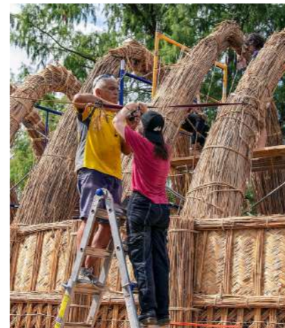
Figure Rd12: Mudhif house arch construction Source: https://www.texasmonthly.com/style/mudhif-houston-rice-university-iraqi-marsh-arabs/
