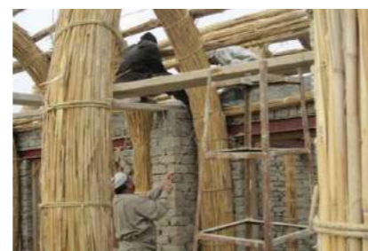
Figure Rd13: Mudhif house arch construction Source: https://www.atlasobscura.com/places/mudhif-houses
