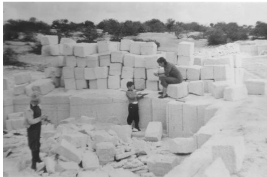
Figure Ss15-16: Cutting coquina blocks from a quarry Coquina shell blocks Source: https://www.sharkbay.org/
