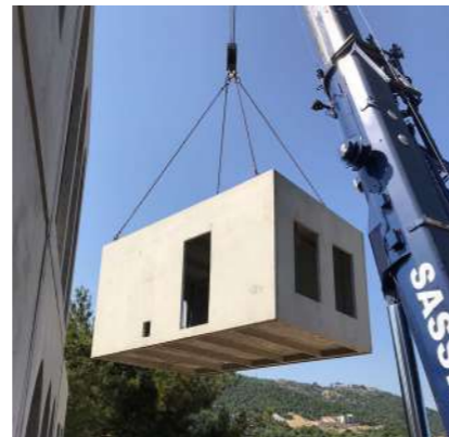
Figure 02.4.2: Concrete modular construction Source: https://megaprefab.com/
