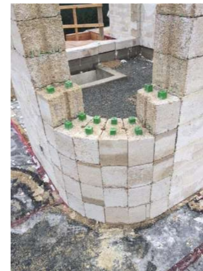
Figure Pf27-28: Just BioFiber - Harmless Home project - building blocks - construction process Source: https://justbiofiber.com/projects/
