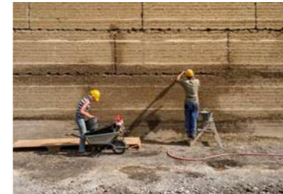
Figure 02.3.3: The Ricola Kräuterzentrum in Laufen Switzerland built with prefabricated rammed earth panels. Project by the architects Herzog & de Meuron and Martin Rauch. Source: https://www.archdaily.com/634724/ricola-krauterzentrum-herzog-and-de-meuron
