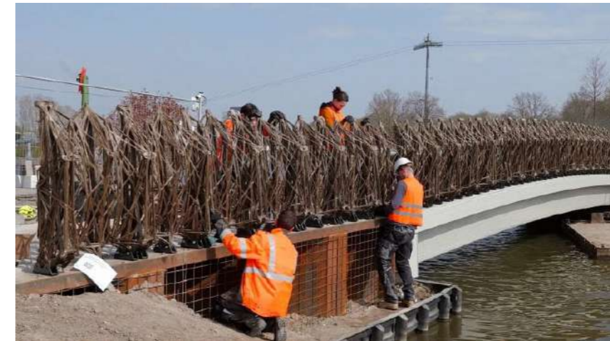
Figure Pf21-22: Smart circular bridge - (NL) - handrail made of robot-wound flax composite filament Source: https://www.dezeen.com/2022/05/05/smart-circular-bridge-flax-completed-the-netherlands-architecture/
