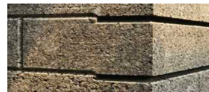
Figure Ck16: Cork house - by Matthew Barnett Howland with Dido Milne and Oliver Wilton - cork blocks Source: https://www.archdaily.com
