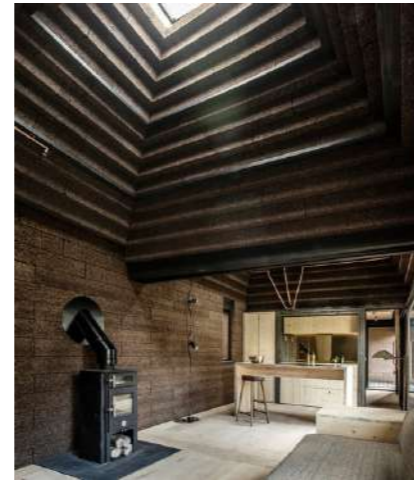
Figure Ck13-14: Cork house - by Matthew Barnett Howland with Dido Milne and Oliver Wilton. Source: https://www.matthewbarnet-howland.com/cork-house
