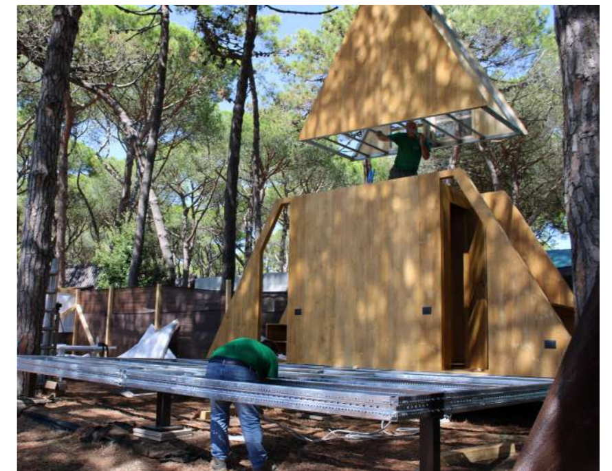
Figure 05.5.6-10: Images of the installation of the prefabricated bathroom and dressing room module Source: Pictures taken by the author of the thesis
