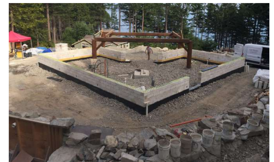
Figure Pf29: Just BioFiber - Serenity Home project - building blocks - construction process Source: https://justbiofiber.com/projects/
