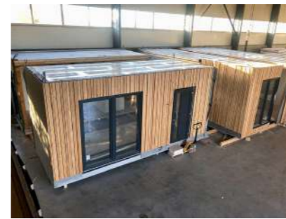
Figure 02.4.3: Wood modular construction Source: https://www.sipeurope.eu/en/se-sip-construction-system/using-sip-system/modular-buildings/
