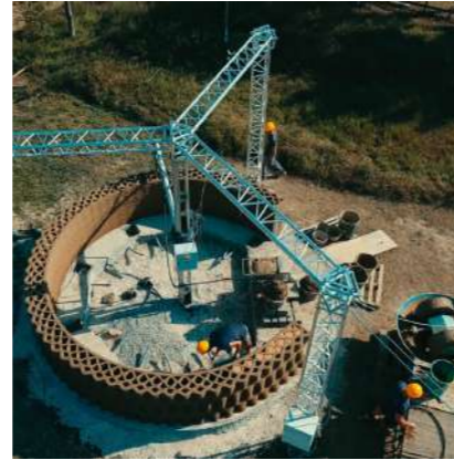
Figure Hk17-18: Gaia project and 3D printing construction process - by Rice House Source: https://www.ricehouse.it/
