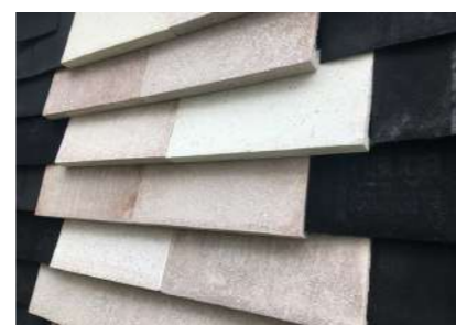
Figure Ss08: Oyster hanging tiles Source: https://localworksstudio.com/projects/shellcrete-transforming-sea-shells-into-low-carbon-materials/
