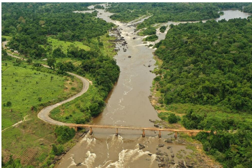
Figure 13: Kikot Hydroelectric Scheme 149
