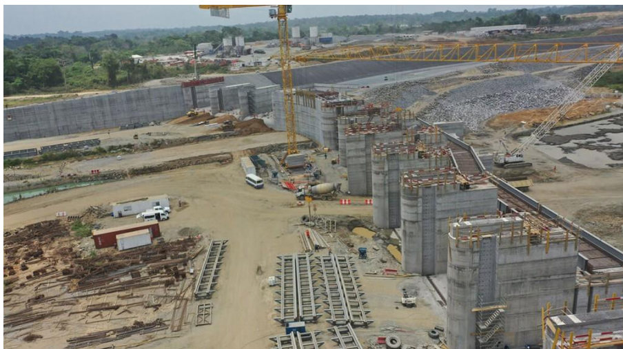
Figure 12a: 148 Dam under construction: Channel intake, spillways, and temporary diversion – April 2022
