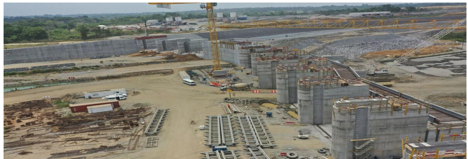
Figure 12a: 167 Dam under construction: Channel intake, spillways, and temporary diversion – April 2022
