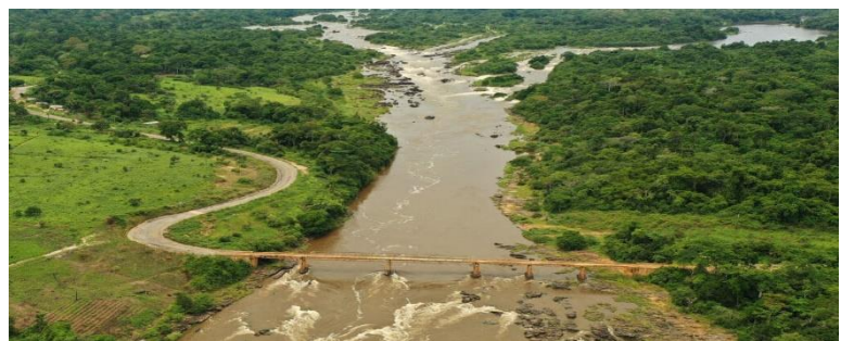
Figure 13: Kikot Hydroelectric Scheme 168
