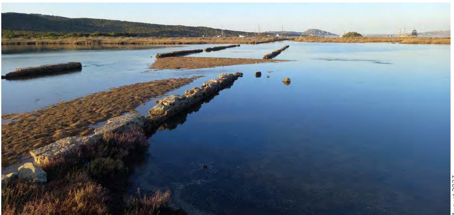
First canal of the Bonifica with concrete borders, used to link Porto Liscia beach with the "La Peschiera" basin
